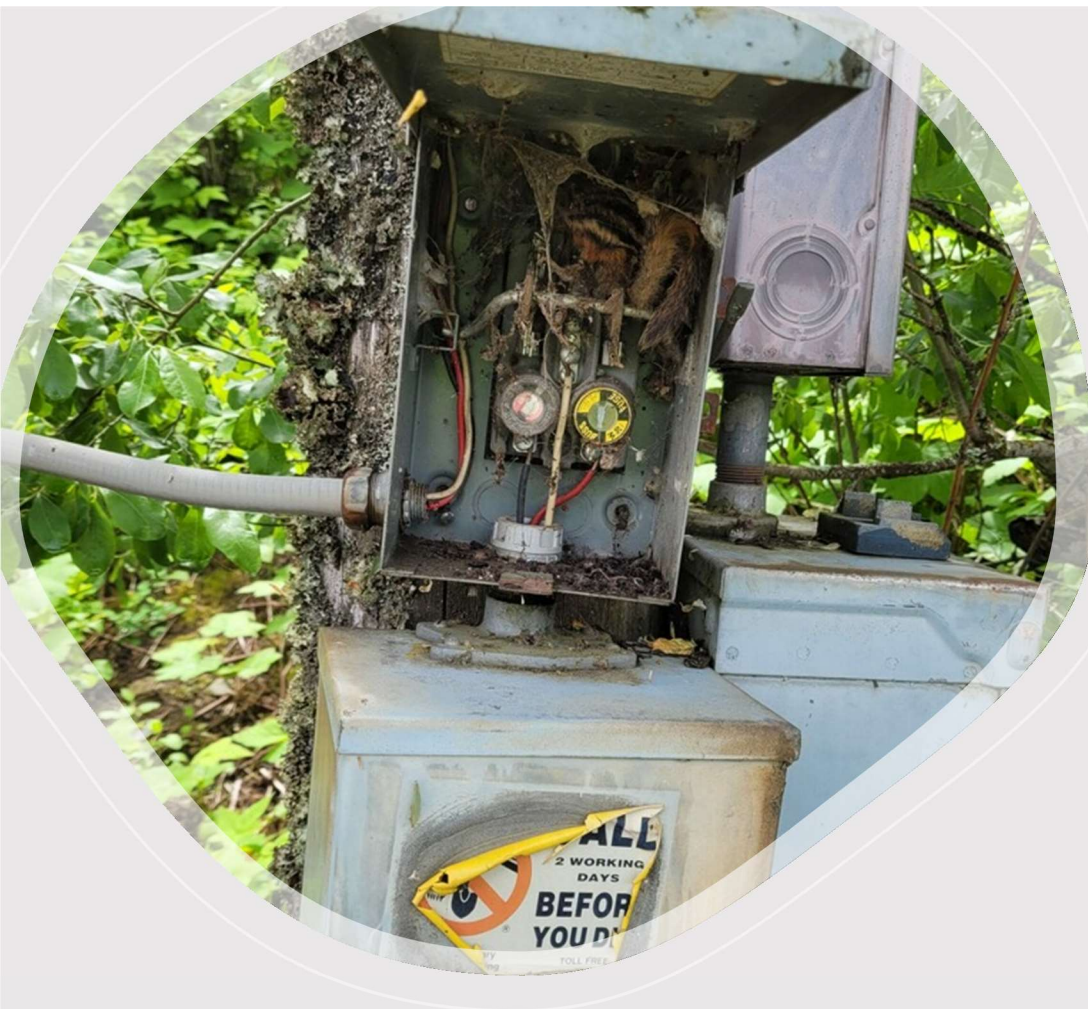
Electrical Service Panels Currently Running Mission Critical Lift Stations 220V 48 AMP
